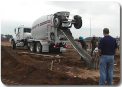
Concrete Redi-mix Truck
